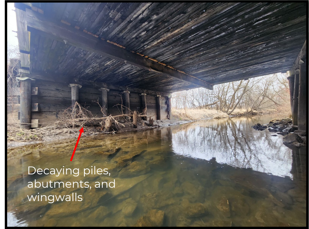
View of Substructure – existing bridge
