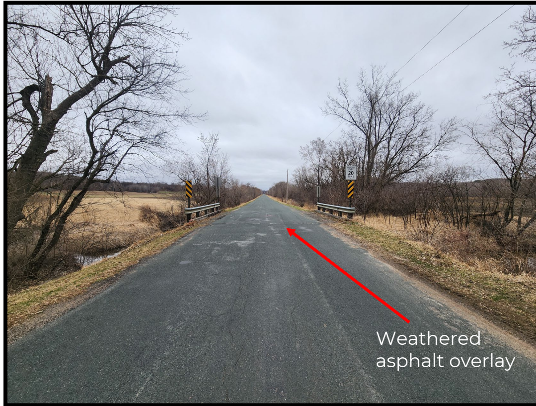
Existing conditions – West Boundary Road
