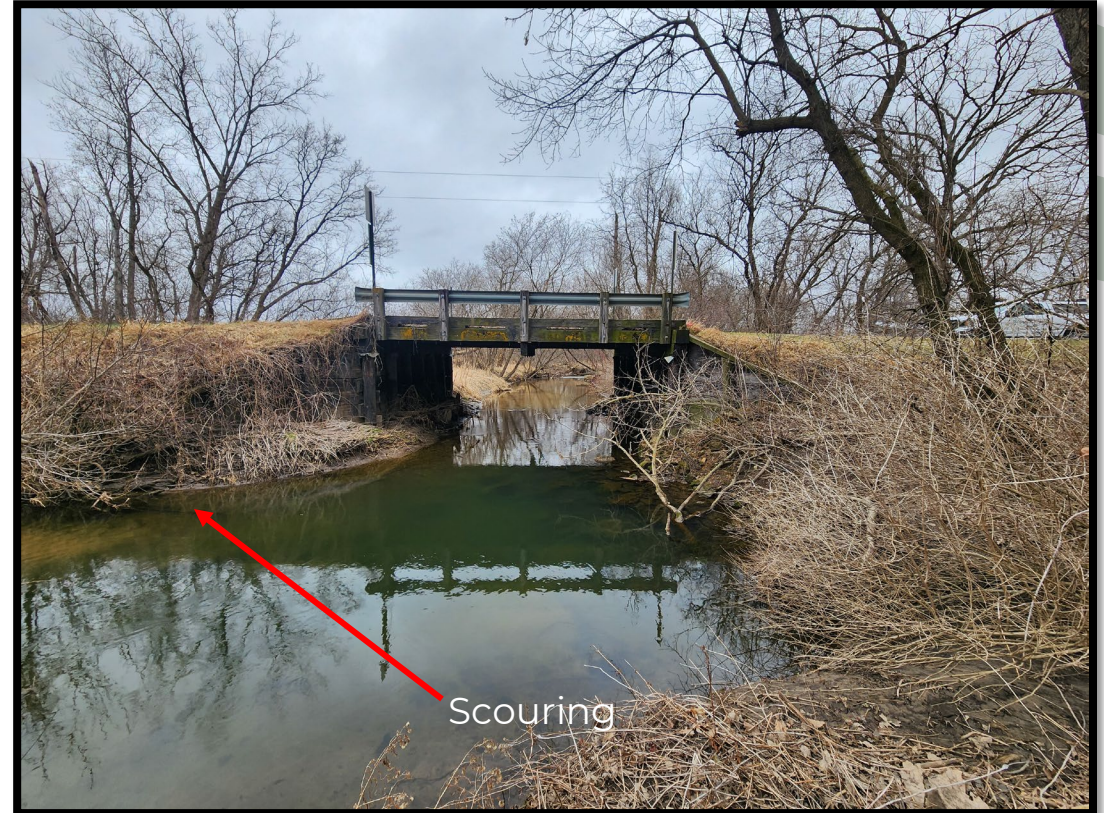
Existing conditions - Sandy Creek Bridge
